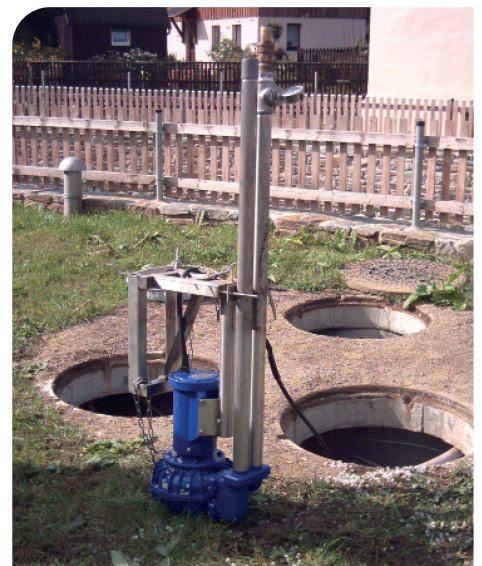
Installation of TMV
